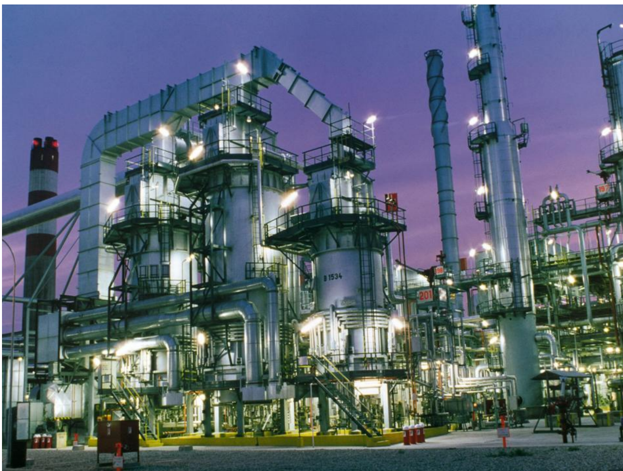
Oil Refinery Plant
