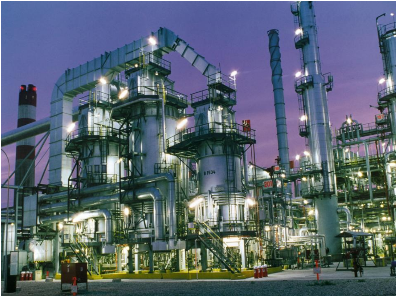
Oil Refinery Plant
