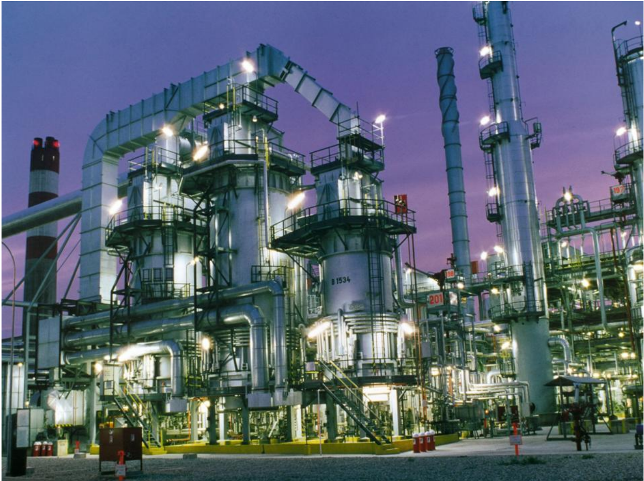
Oil Refinery Plant
