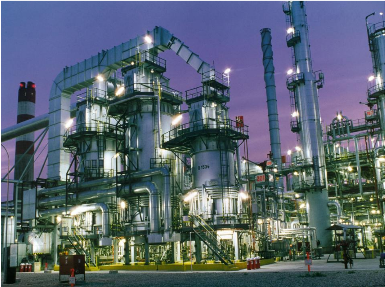
Oil Refinery Plant
